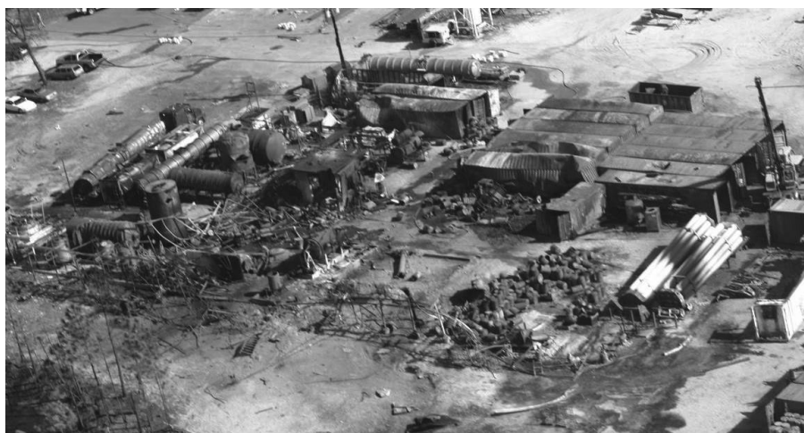
Aerial photograph of T2 taken December 20, 2007. (Courtesy of Chemical Safety Board.)
