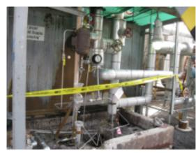
service. Not long after the valve was opened, the tubing directly downstream from the valve came apart. The tube is pressurized during the alkylation process and there was insufficient tightening between the tube and compression joint allowing the tube to be forced off.
