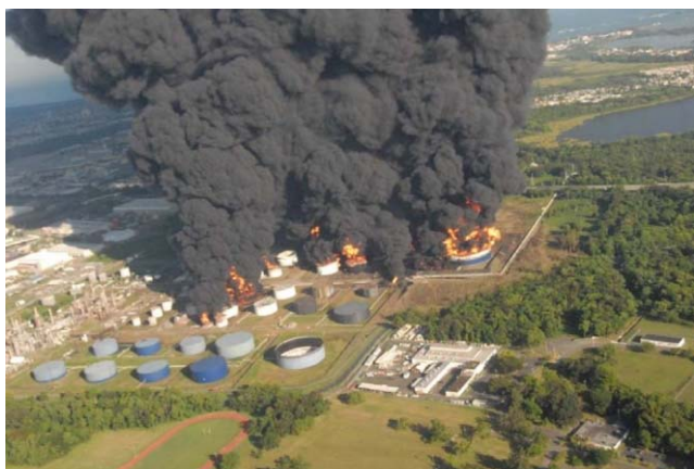
Multiple tanks burning in the fire
