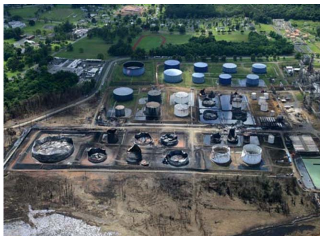
Damage to the facility after the fire
