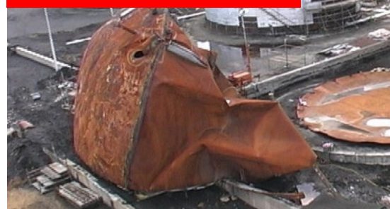
Fig. 2: Hot oil tanks
