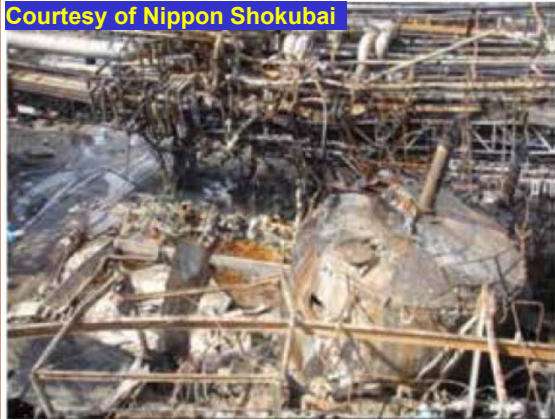
Photo 1: Destroyed AA Tank
